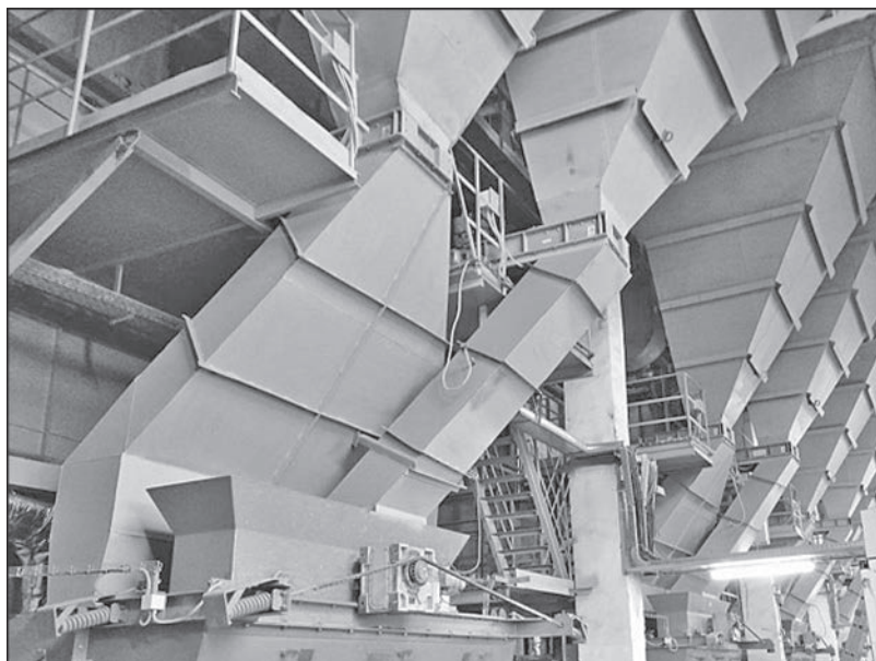
Fig. 8.8. “Radiant” boilers at the Khorostkiv Sugar Plant, retrofitted for burning biomass pellets and/or gas coal
