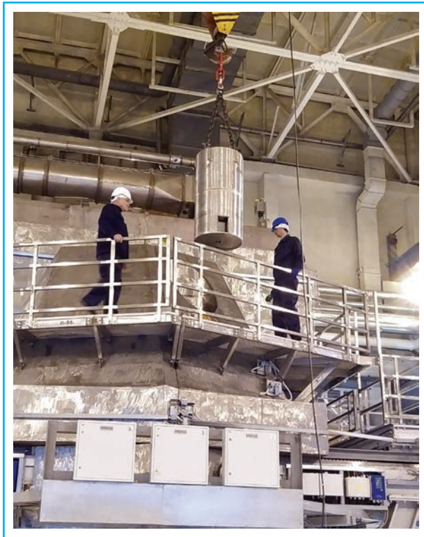
Building of the nuclear subcritical installation “Neutron source”
